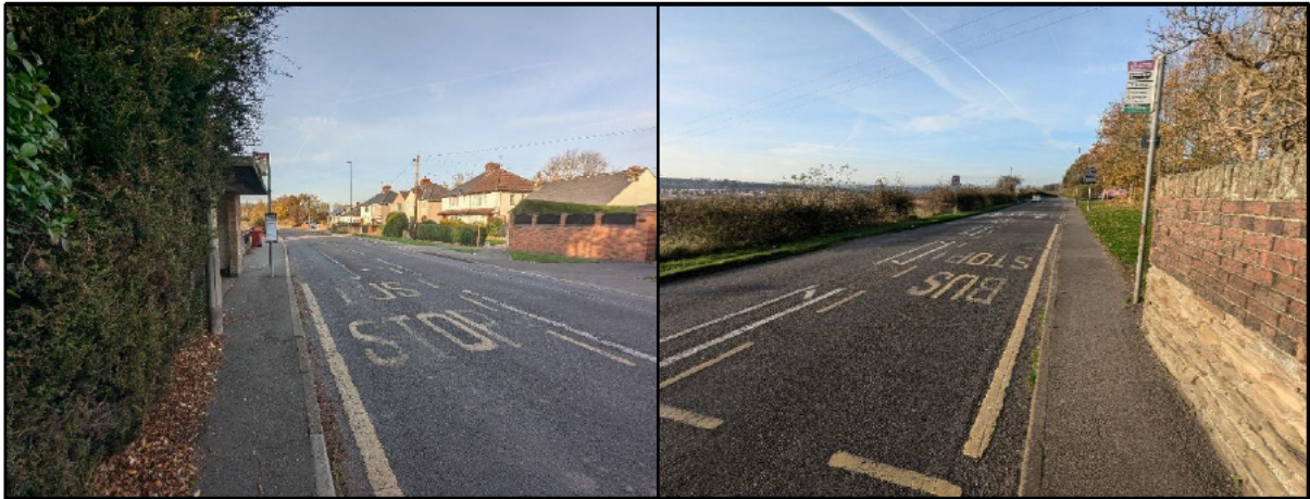
Figure 3.5: A632 Top Road Bus Stop
