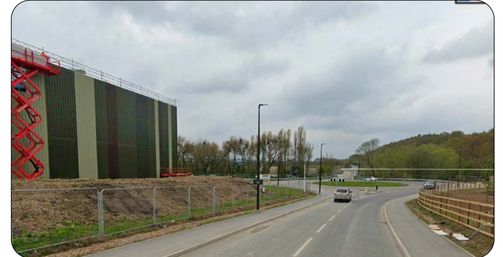
Photograph 11: Showing cladding and vegetation at the former Coalite site, Horizon 29
