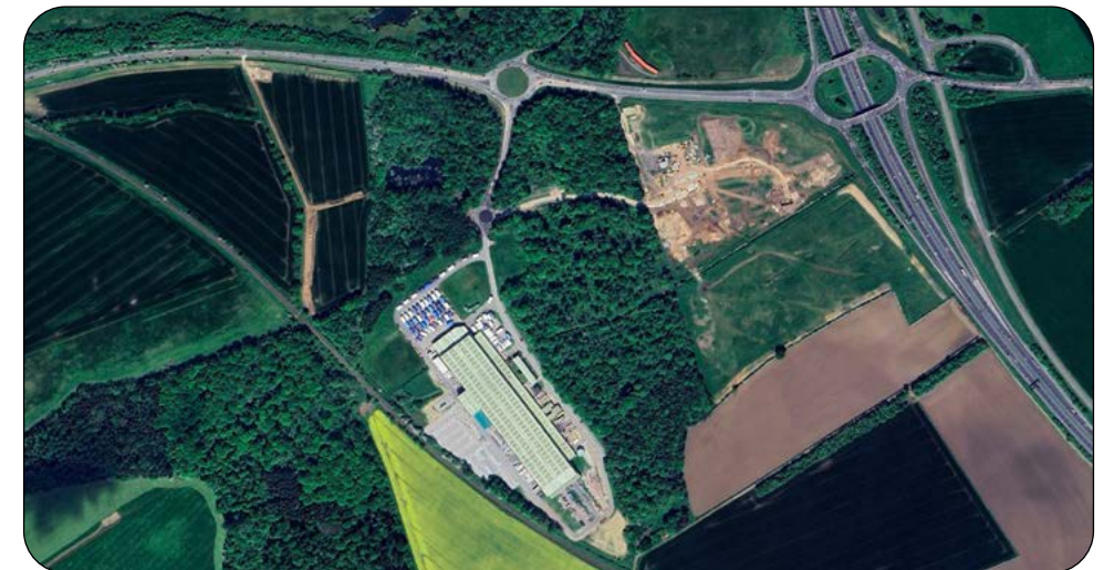
Photograph 13: Aerial view showing Harrogate 47 site off the A1 and A59, Flaxby & Shepley Spring, Knaresborough
